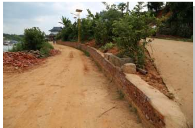
Mud-slide preventing wall and solar energy-saving lamp
